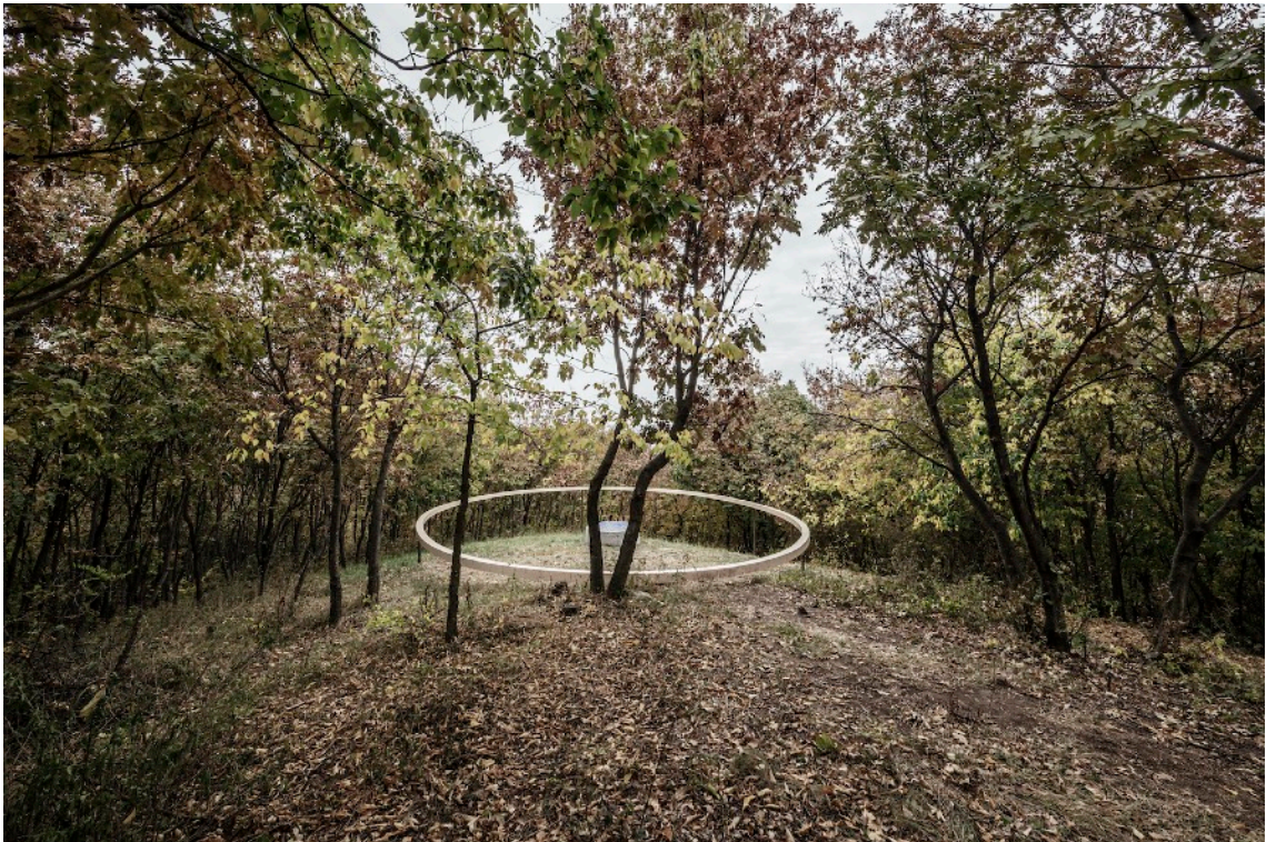
Kázmér Domokos, Eszter Kaderják, Dorottya Kéry, Anna Pongrácz, Noémi Éva Sebestyén, and Biborka Kelemen: Forest Chapel, Pannonhalma (2018). Community-built work. The 14 x 7 m oval shape is made of wood and iron, while the central altar is made of concrete and covered by glass mosaic.
