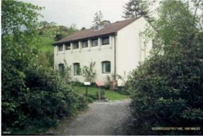
Center for Alternative Technology (CAT) Machynlleth, Wales, UK Eco-house, (whole house) 1976 Foto: Szekér László, 1986
